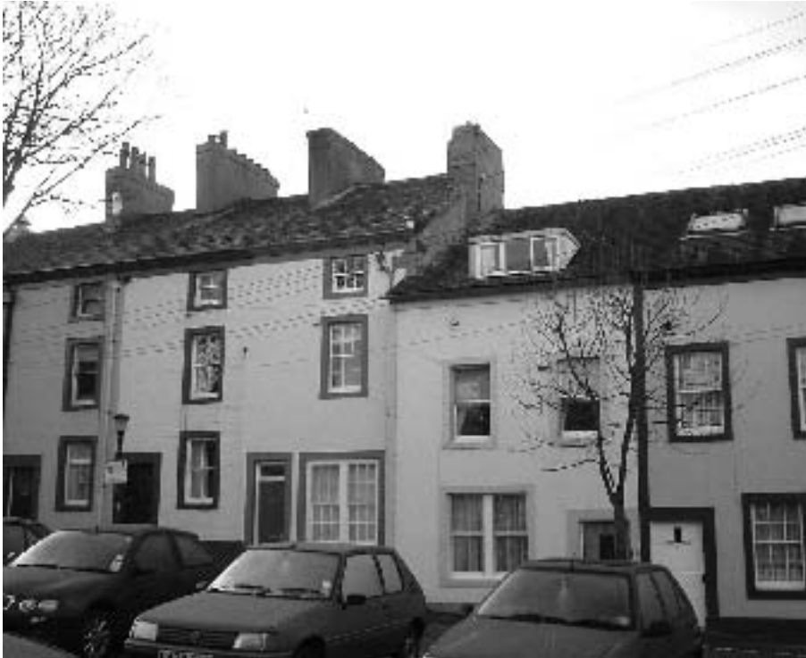
Portland Square, Workington
